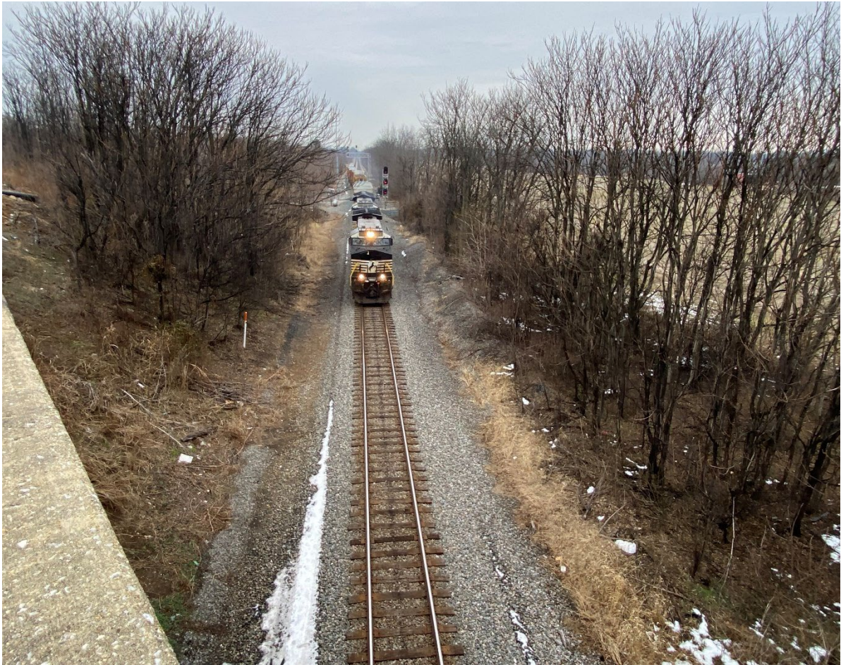
Figure 7: Norfolk Southern Railroad near WV Route 9
