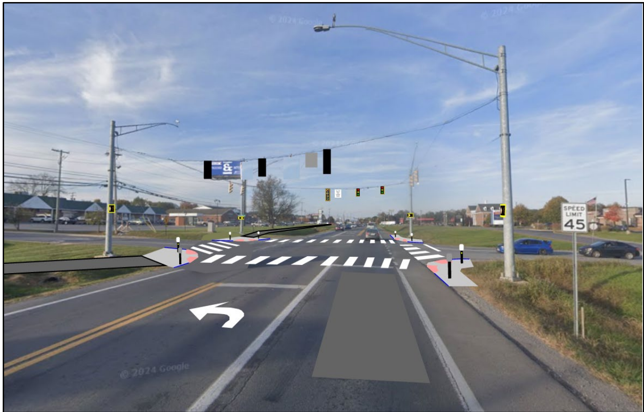
Figure 16: Typical Pedestrian and Flashing Yellow Arrow Improvements at Signalized Intersections along Edwin Miller Boulevard
