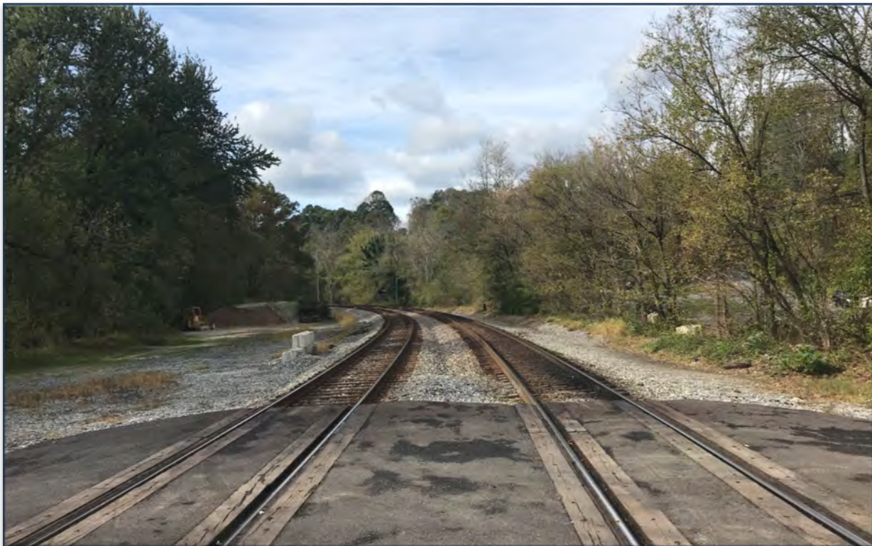
View looking West of CSX Railroad from Current At-grade Crossing
