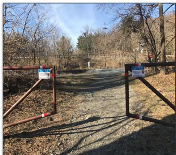
Current Lockable Gates at the Weverton Crossing
