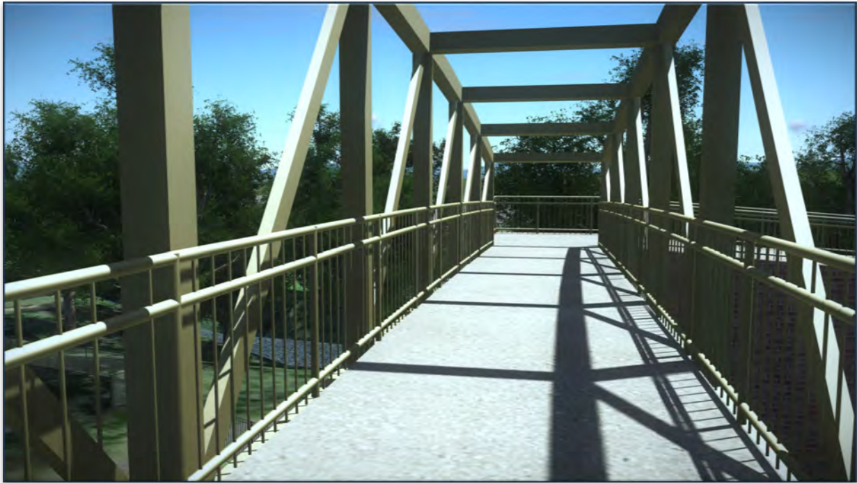
Figure 15: Close-up View of Pedestrian Bridge Span
