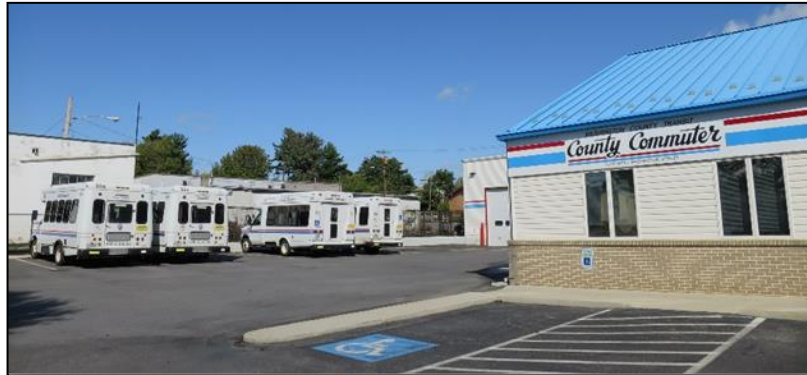
Figure I-25: Washington County Transit Administrative and Vehicle Maintenance Facility
