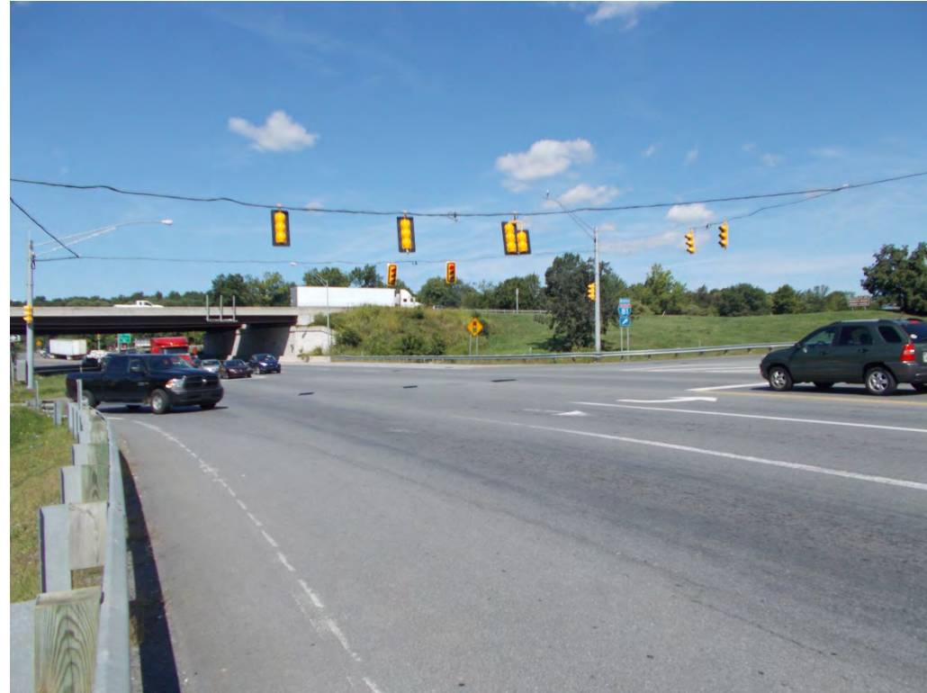
View Westbound on WV 45 at I-81 NB Intersection
