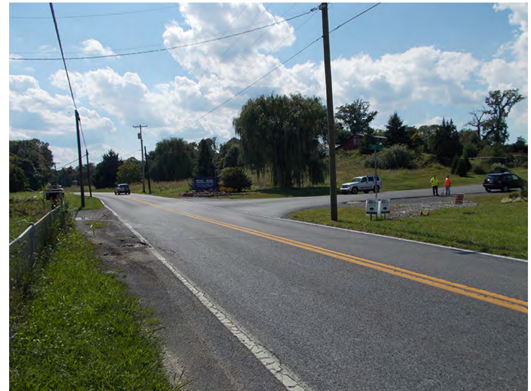
View Westbound along WV 45
