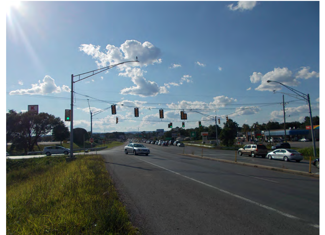
View Westbound along WV 45
