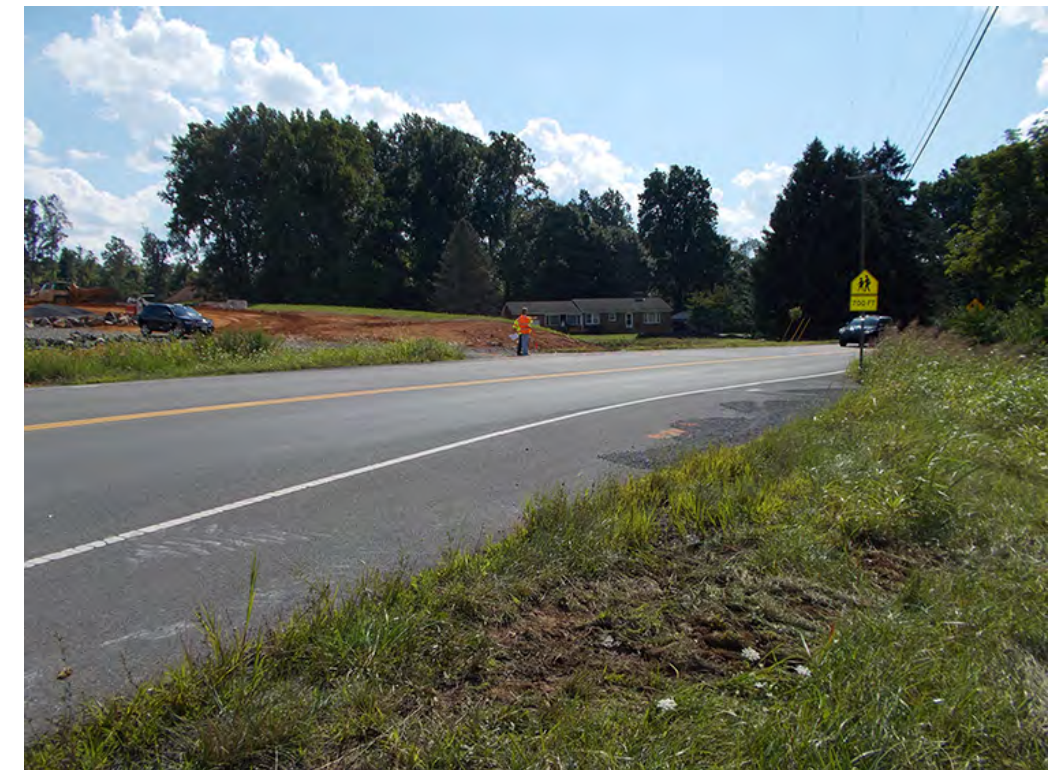
View Westbound along WV 45
