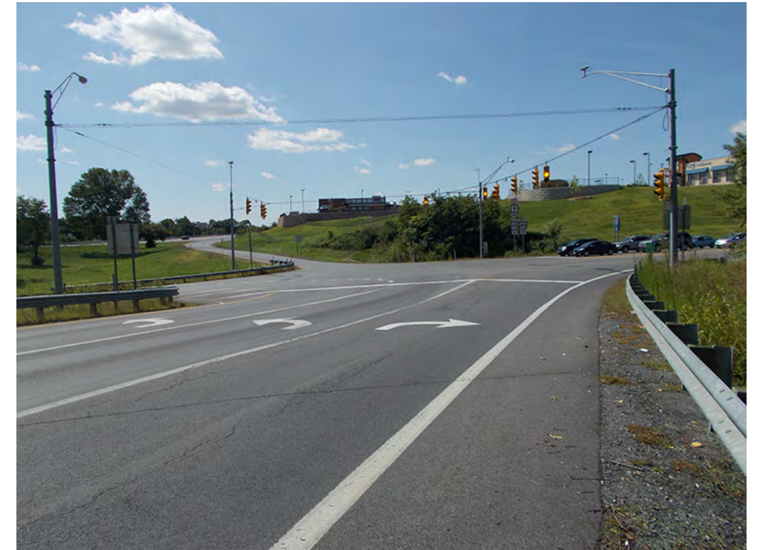
View Southbound on I-81 Southbound off-ramp
