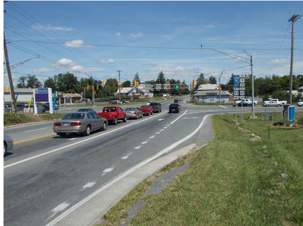
View Northbound along Winchester Avenue
