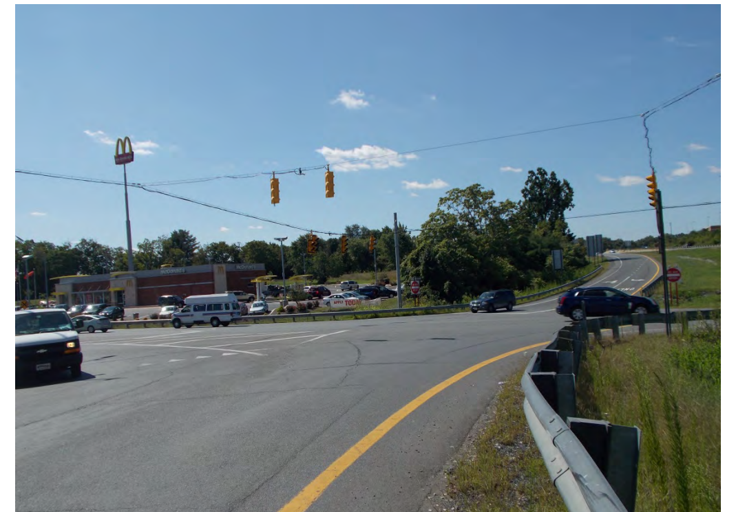
View Southbound along I-81 on-ramp back towards WV 45
