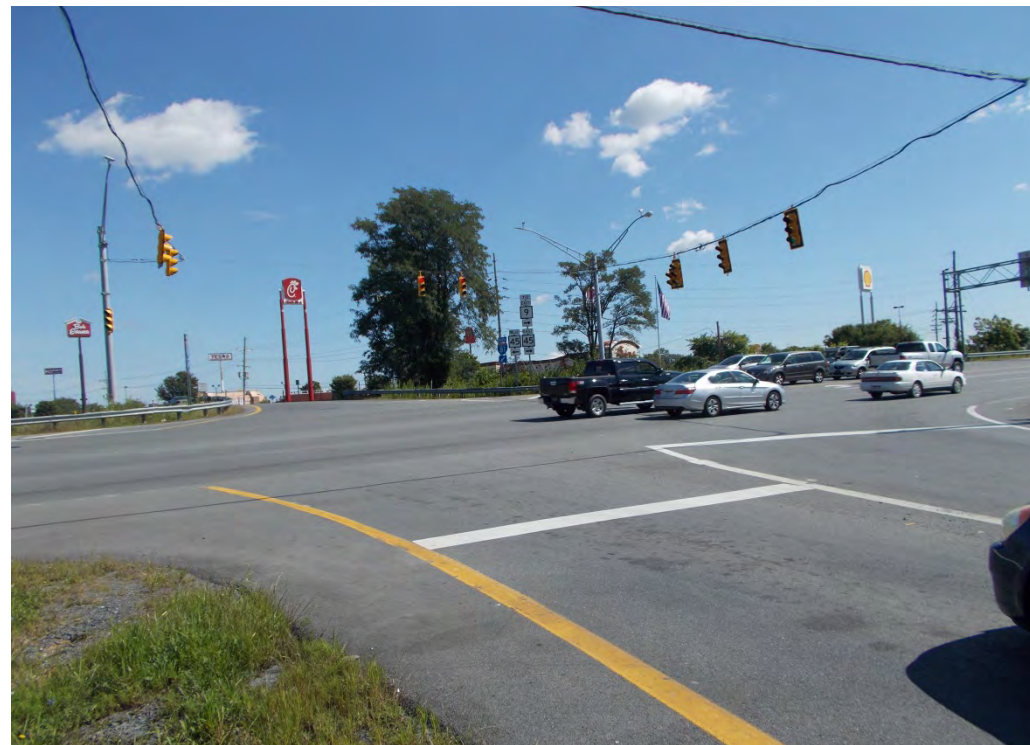
View Northbound along the I-81 NB off-ramp at WV 45
