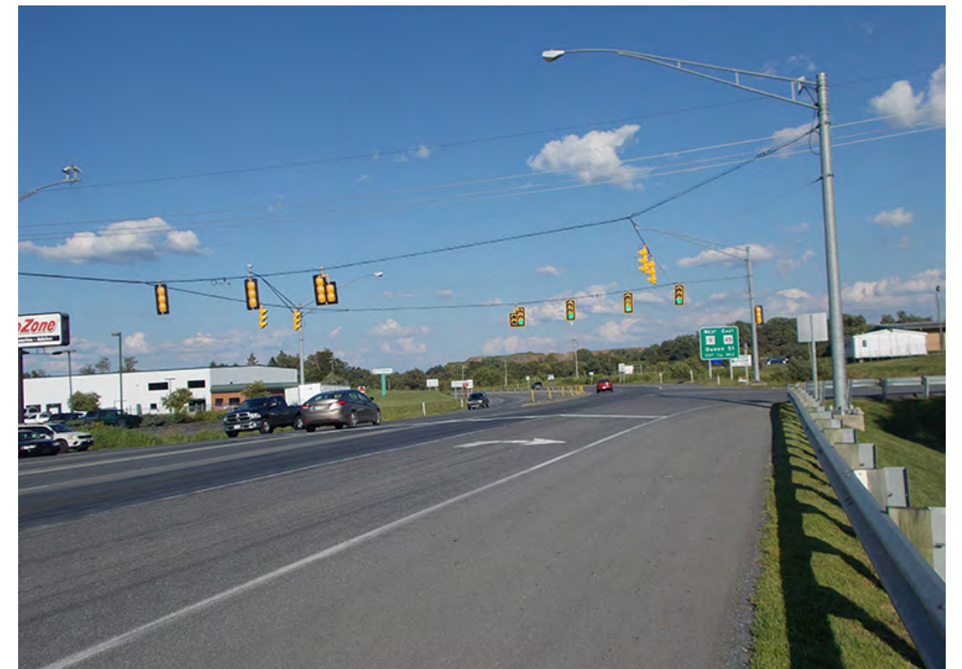
View Eastbound along WV 45.
