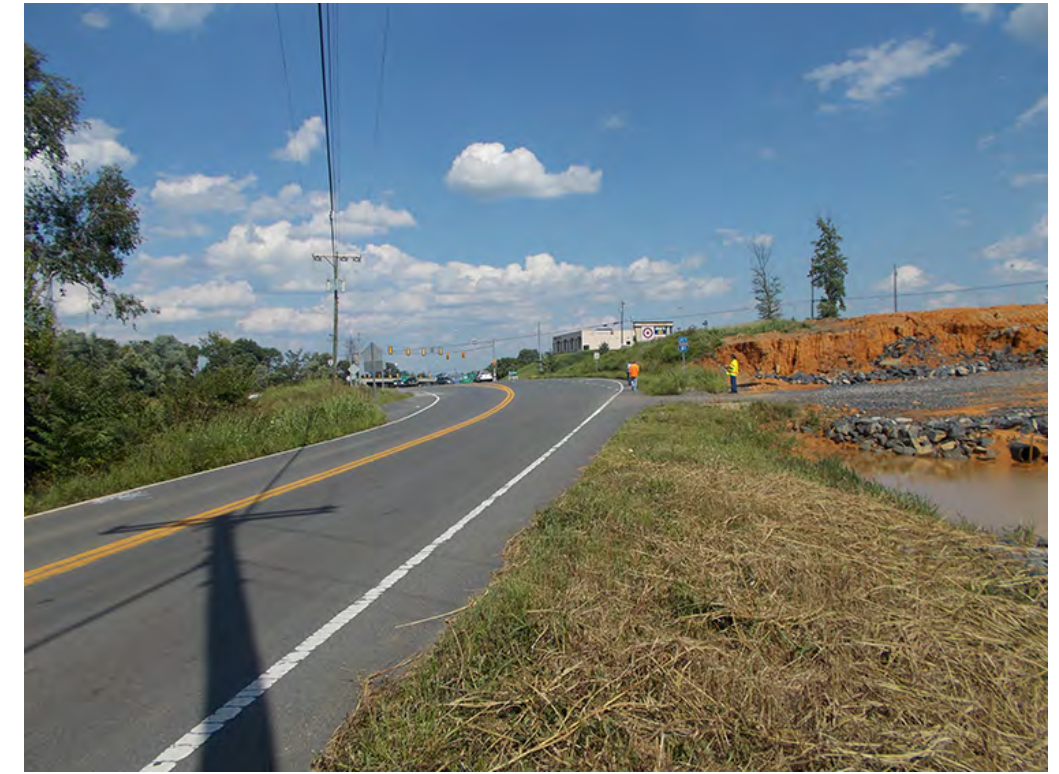
View Eastbound along WV 45
