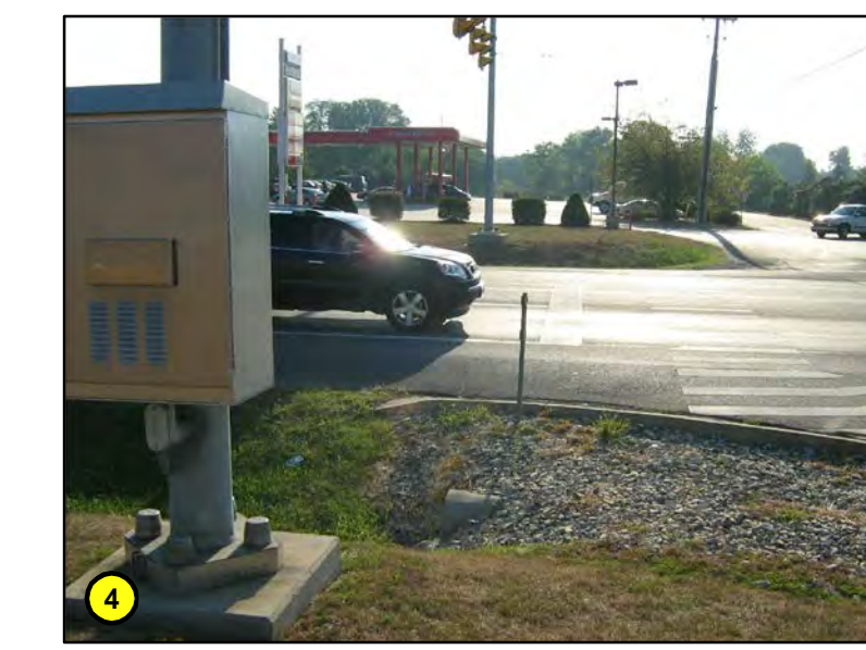
Crosswalk at Sheetz Intersection: The lack of connecting sidewalks and crosswalk signalization contribute to a dangerous environment for the pedestrian. Striping for the crosswalk is the only indication this is a pedestrian route.
