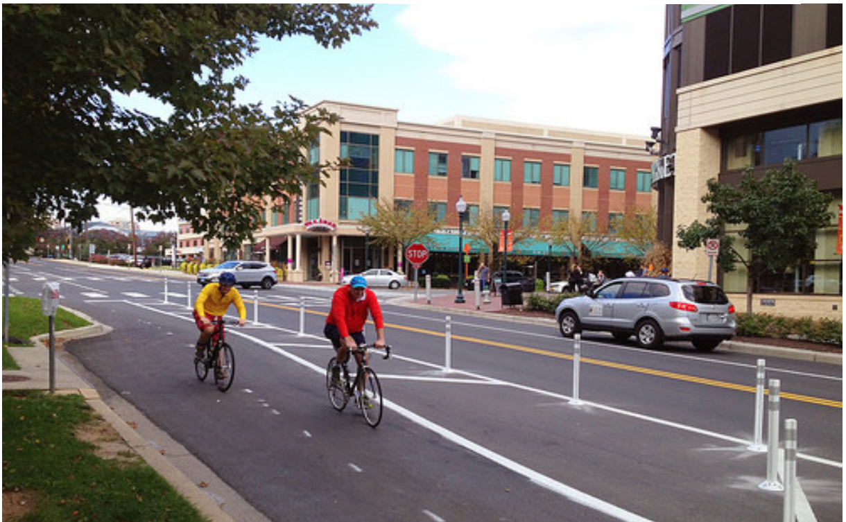
On-way protected cycle track on the left is separated using marking, flexible delineator post at Woodglen Drive cycle track (photo from GGW)
