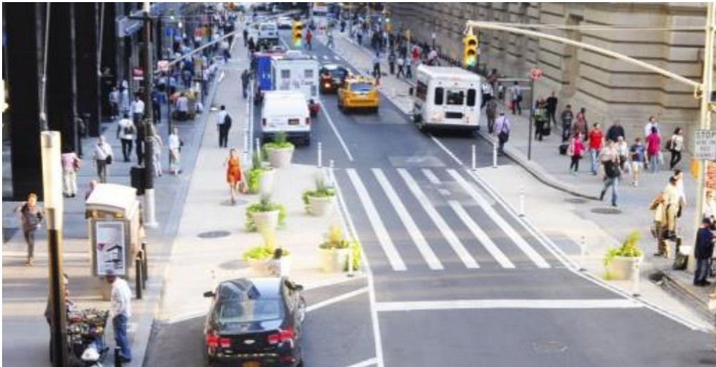
Curb extension at mid-block crossing in New York (Photo: NACTO)
