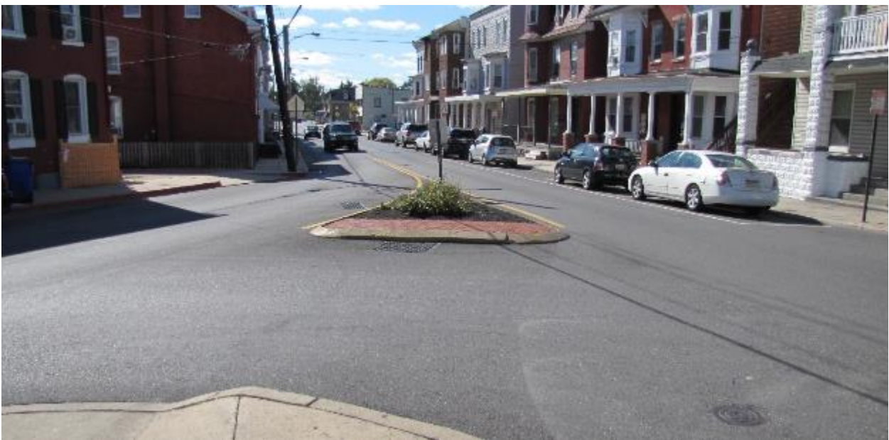
Lack of crossing marking or signage at Potomac Street and Locust Street can be a potential safety risk.
