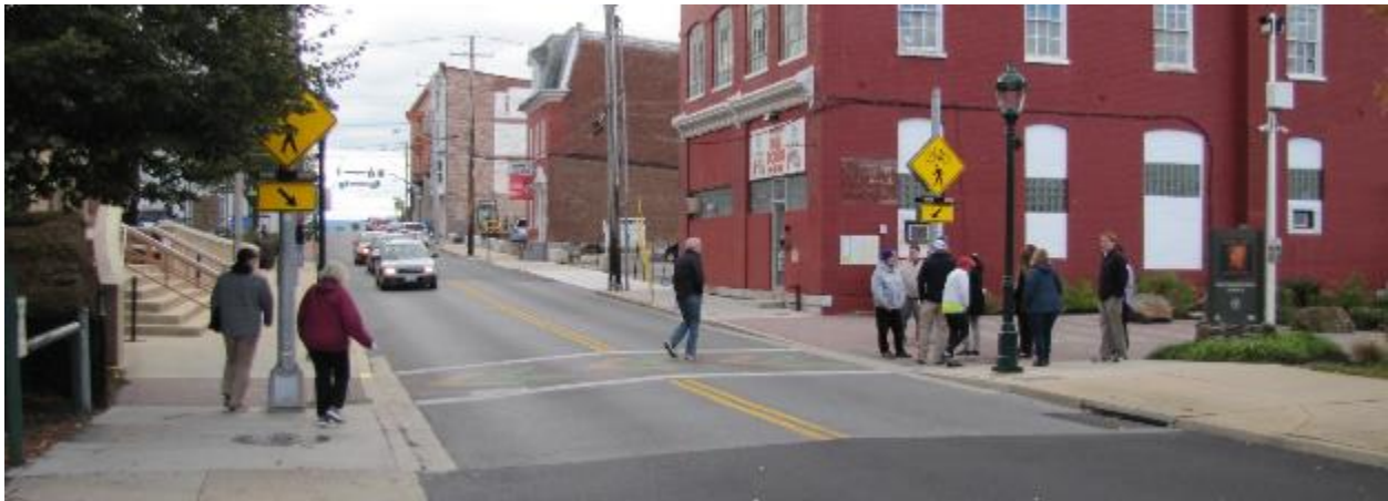
A midblock crossing with high visibility and RRFBs connects two sides of Cultural Trail at Antietam Street.
