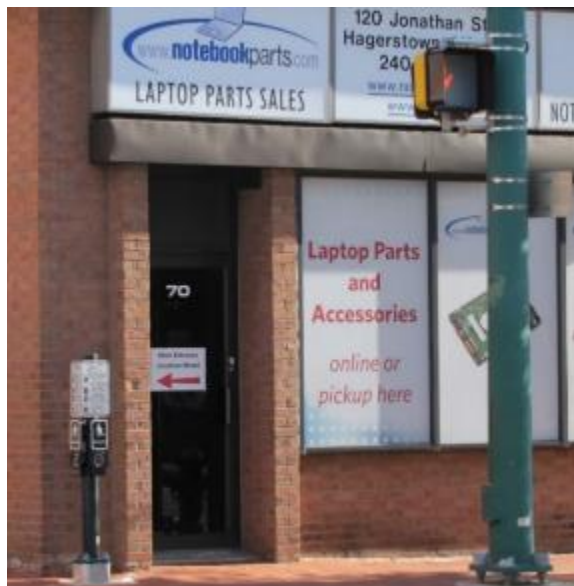
The pedestrian push buttons at Franklin Street and Jonathan Street are co-located and do not have an audible notification to pedestrians.
