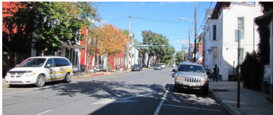
Potomac Street shifts from two lanes to one lane between Lee Street and Sycamore Street.
