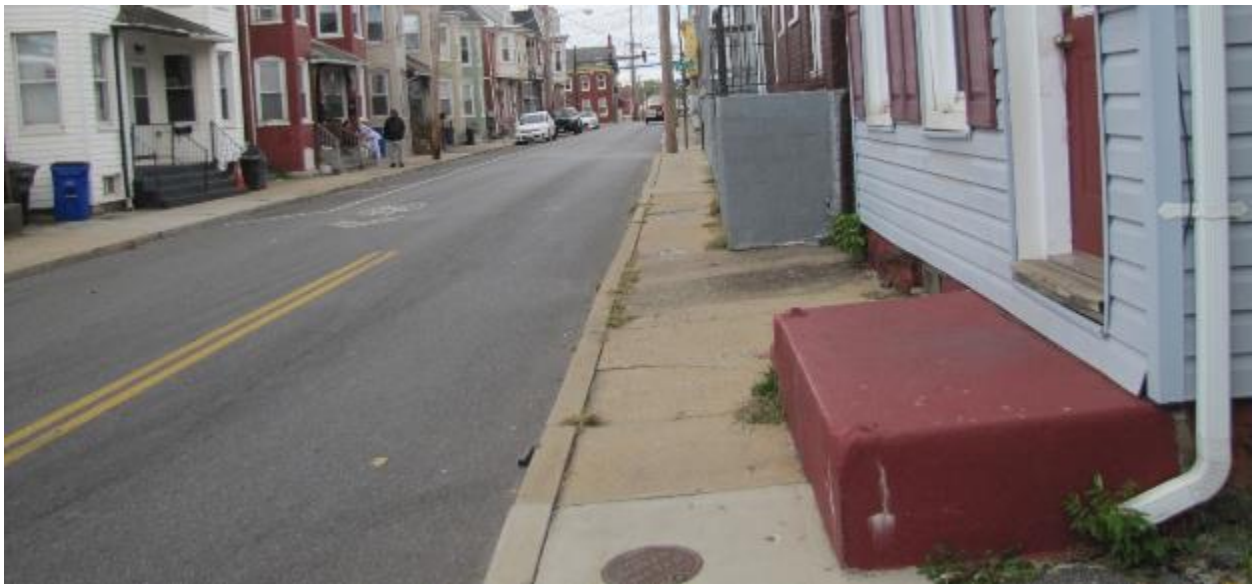
Residential stoops encroach on the sidewalk, narrowing space for pedestrians (Lee Street between Locust Street and Potomac Street).
