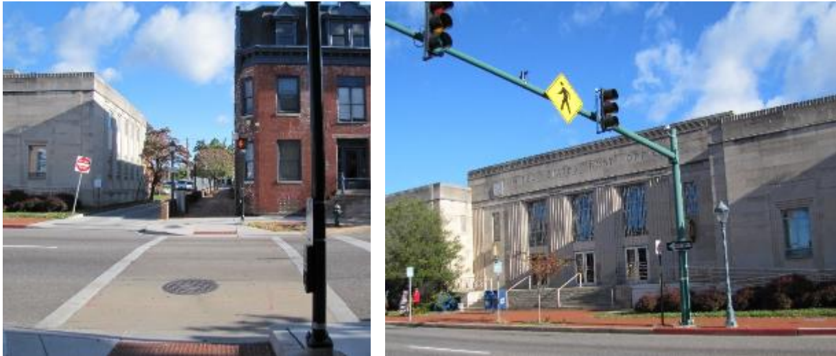
On Franklin Street, there is a signalized mid-block crossing in front of the Post Office (between Jonathon Street and Potomac Street).
