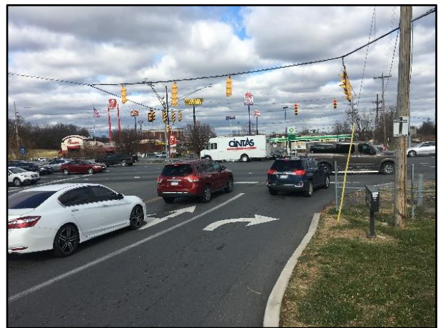
Right: The intersection of Foxcroft Ave and Apple Harvest Drive; it is a busy intersection with many turning movements, and there is no pedestrian signal phase or crosswalks.
