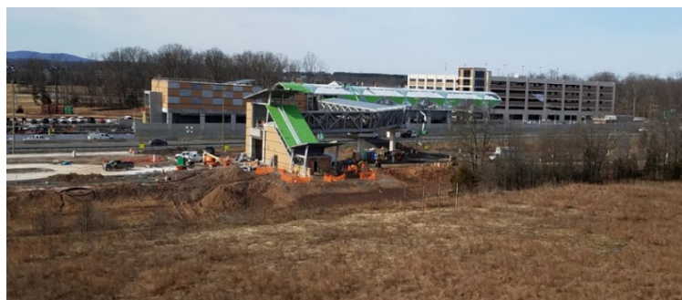
Construction at the Ashburn Metro Station
